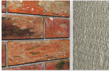
Wall to wall construction joint
